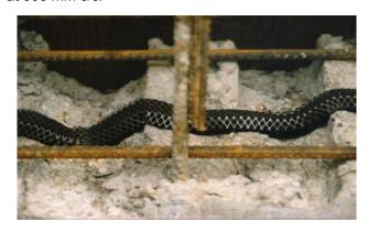
End-to-end or end-to-side junctions are created by simple butt joints. Ensure continuity is achieved through Revofix Mesh, by pressing ends firmly together. Start at junctions; do not stretch Waterstop RX101 to fit. Do not overlap the Waterstop RX101.
